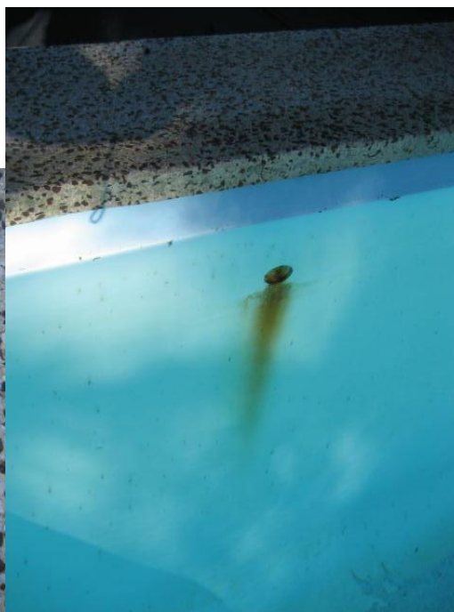
Filter outlet rust stained
