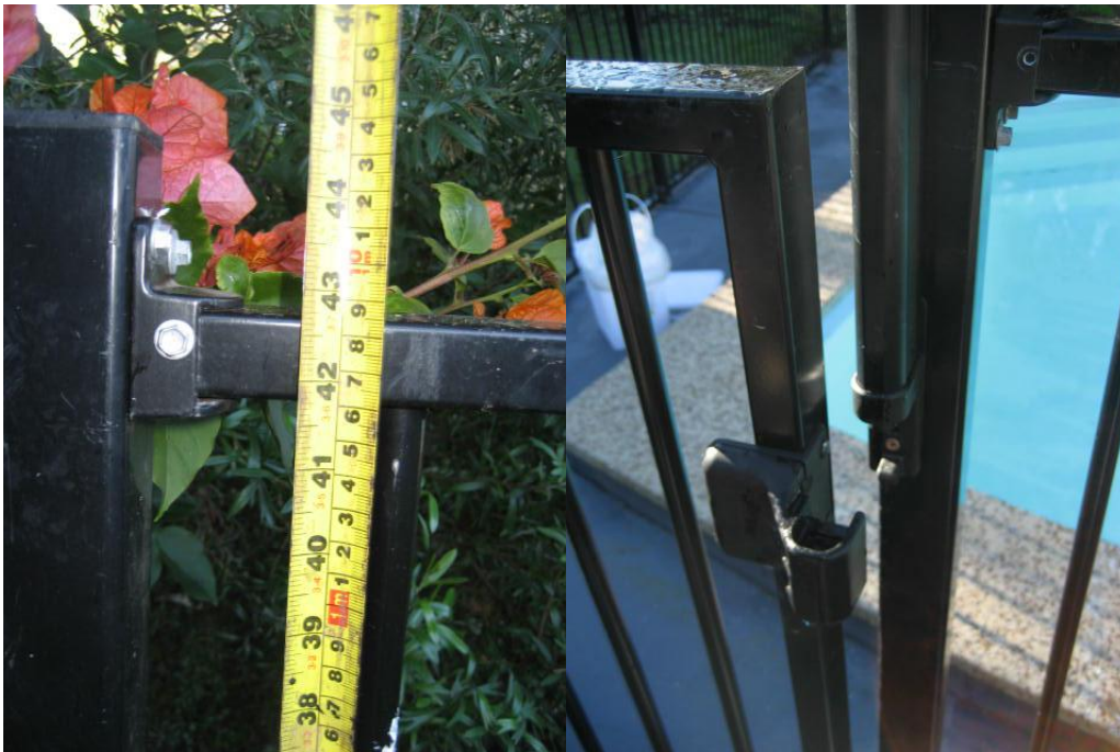
Pool fence is less than 1200mm high by 115mm
