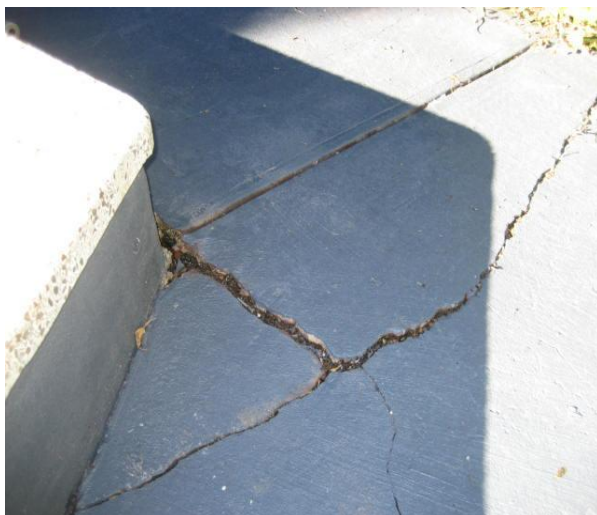
Cracks in concrete paths surrounding the pool may be a trip hazard
